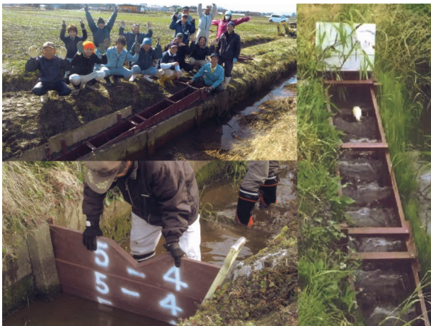
Installing fishway using FFU remnants and observing running-up fish
